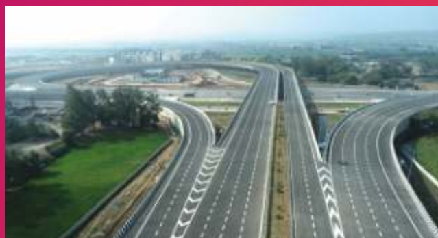
YAMUNA EXPRESSWAY: 13 KM
